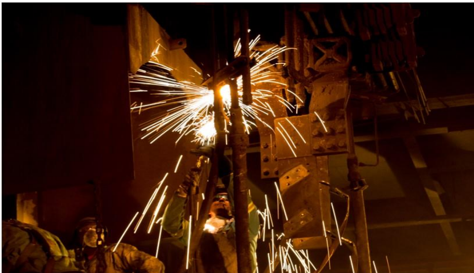
Figure 2 & 3: Dismantling of equipment at the Transalloys site
